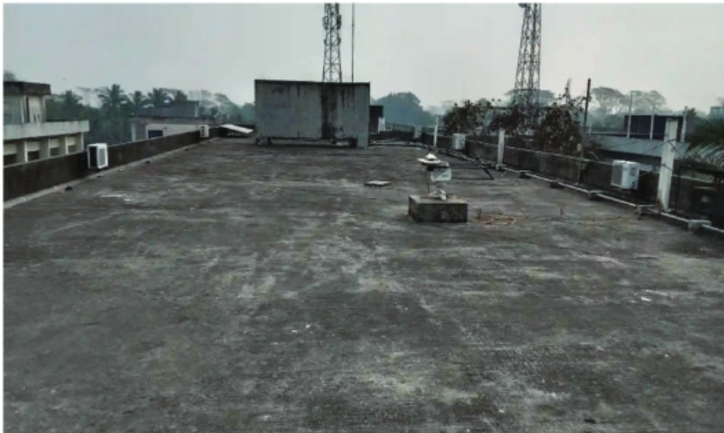
Figure 4. Rooftop view of the academic building for CSE
